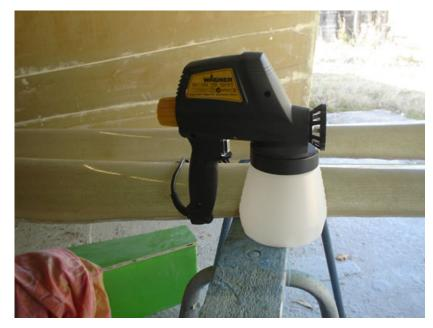
We spray primer twice. After the first coat we sand the boat and fix any imperfections which are only visible after the boat is painted.
