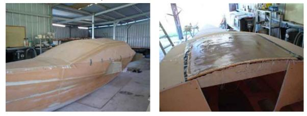
This is a good time to make a hatch top. Plastic is laid over the cabin roof and foam is temporarily screwed down and glassed on the top surface.
