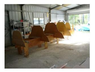
If the boat is to be built using plywood then the sheets are scarfed together and joined to the building frame. The edges bogged and sanded and the glass in laminated over the hull while it is still on the frame.
